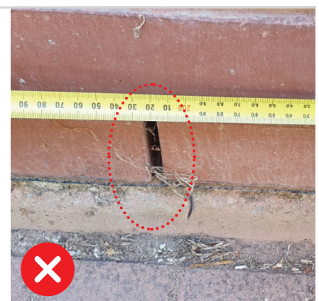
Figure 1.3 The presence of a penetration greater than 5mm in diameter through the non-combustible barrier to a habitable room and within 600mm of the left edge of the battery system is non-compliant unless sealed with fire-retardant material.
