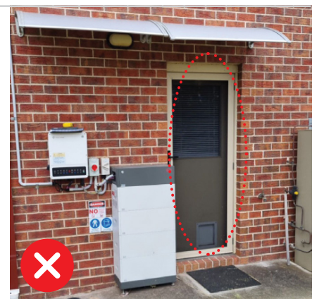
Figure 7.3: This battery system is non-compliant as it has been installed too close to an entry or doorway.
