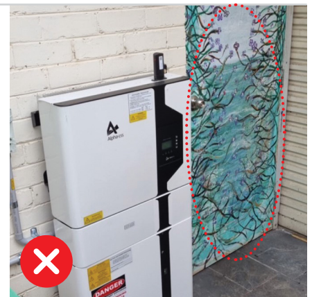
Figure 7.2: This battery system is non-compliant as it has been installed too close to an entry or doorway.
