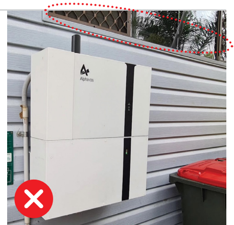
Figure 6.2: In this example the window above the battery system vents a habitable room and is located within the exclusion zone outlined in Figure 6.1.
