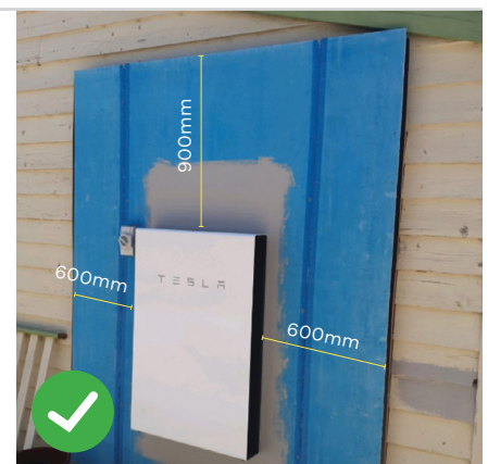
Figure 1.2 In this example a compliant non-combustible barrier made out of compressed cement sheeting has been installed to the appropriate dimensions as laid out in Figure 1.1.
