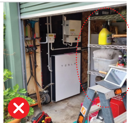
Figure 1.1: Non-fixed shelving is not adequate mechanical protection for a battery system installed in an area accessible to cars.
