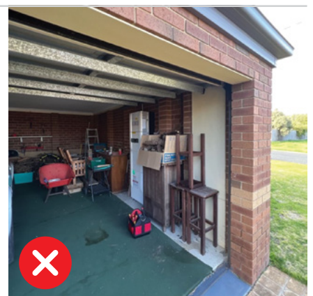
Figure 1.3: A vehicle could enter into this space, meaning that fixed vehicle mechanical protection would be required regardless of any non-fixed objects that could be installed.
